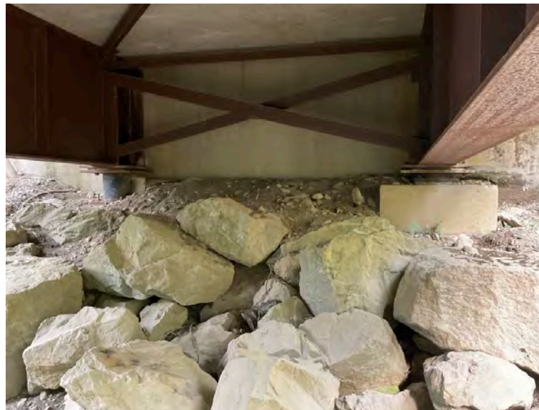
Right Bank Abutment when facing downstream
