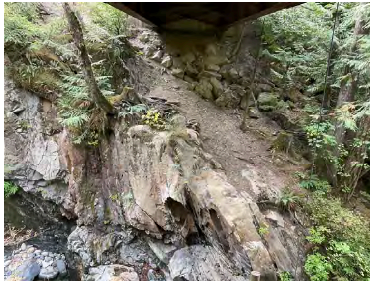
Left Bank Abutment when facing downstream
