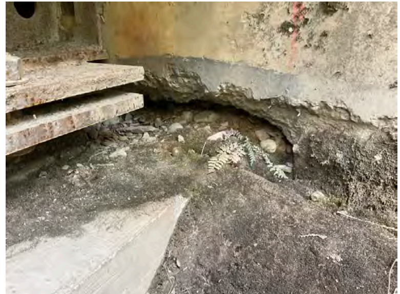
Upstream right bank ballast wall condition
