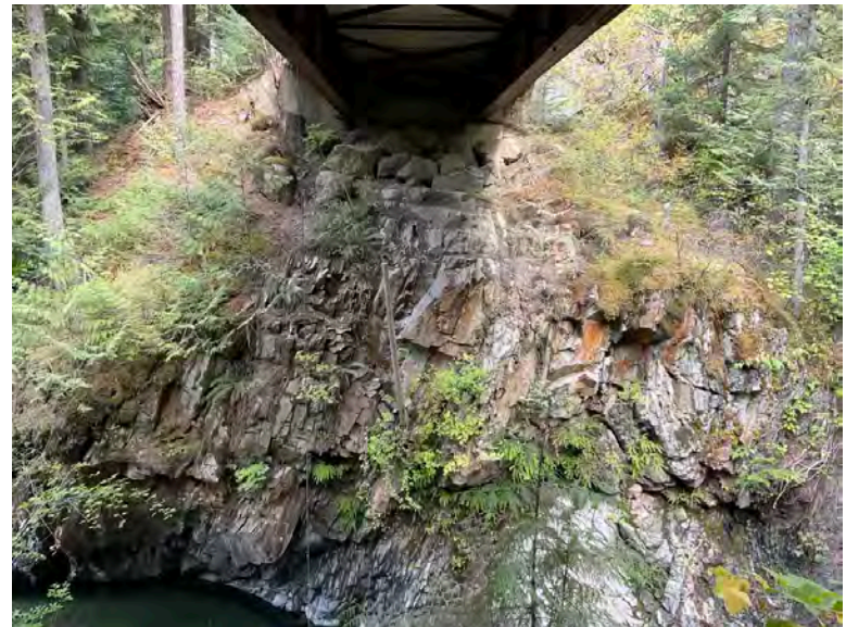
Right Bank Abutment when facing downstream
