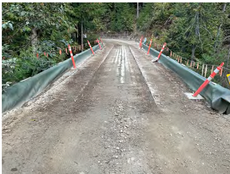
Timber deck placed on top of composite deck
